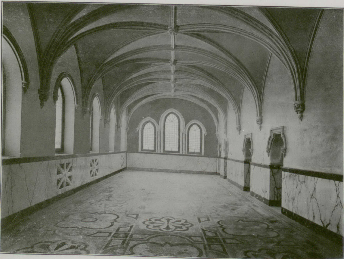
GROUND PLAN AND CREMATORIUM HALL OF CONSERVATORY AND CREMATORIUM, MOUNT ROYAL CEMETERY, MONTREAL.
