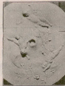
CENTER FLOWER IN STAFF FOR RESIDENCE, ST. GEORGE STREET. By Wm. J. Hynes, Toronto. F. H. Herbert, Architect.
