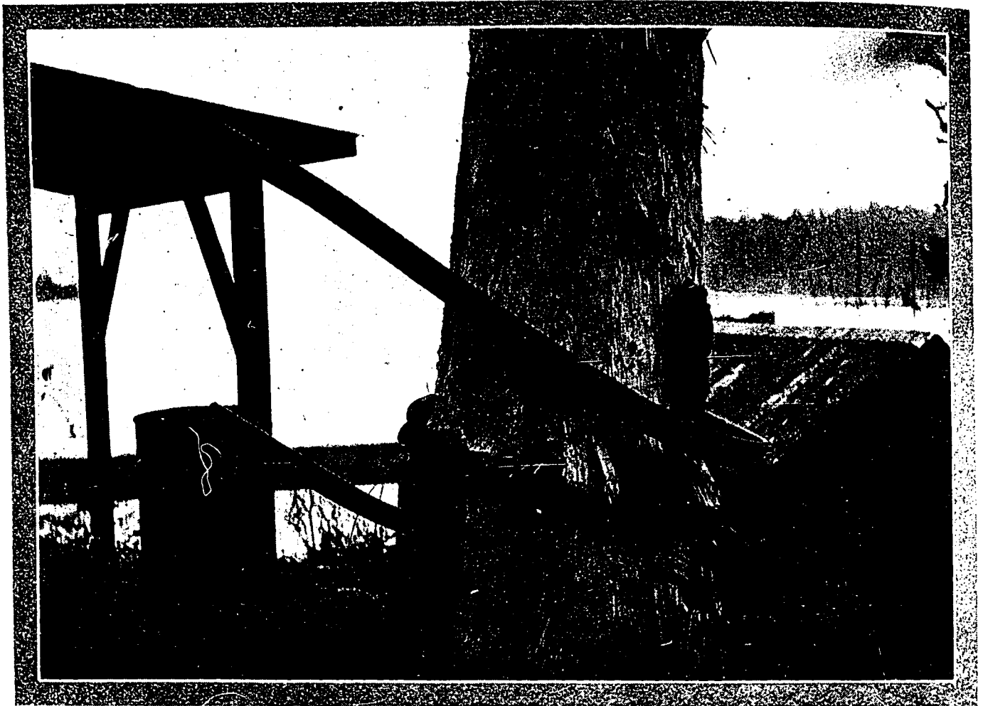
STEEL RAIL, TWISTED AROUND TREE TRUNK BY FORCE OF EXPLOSION
