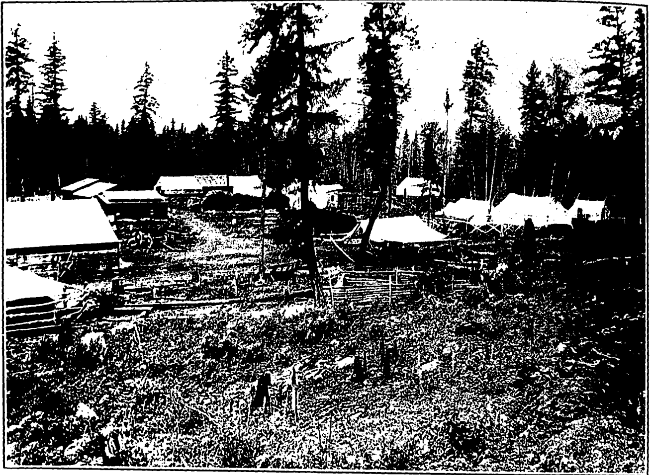
RAILWAY CONSTRUCTION CAMP AT CHU CHUA, B. C.
