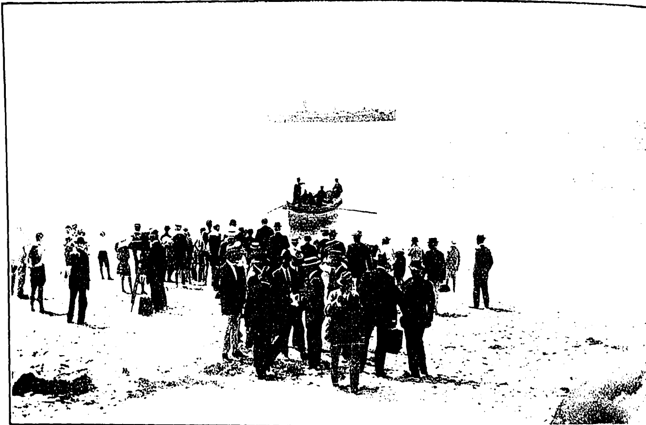
LANDING SHORE END SYDNEY-AUCKLAND CABLE. FIRST BOAT TO LAND ON BONDI BEACH. S.S. SILVERTOWN IN DISTANCE
