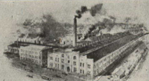
NEW FACTORY BUILT IN 1895 SINCE THEN THE FOLLOWING EXTENSIONS HAVE BEEN MADE MACHINE SHOP LENGTHENED 140 FT NOW 440 x 120 BOILER SHOP 100 FT NEW 220 x 80 WITH CORRESPONDING INCREASE MOULDING SHOP 100 FT NEW 180 x 80 IN EQUIPMENT BLACK-SMITH SHOP 40 FT NEW 100 x 40
