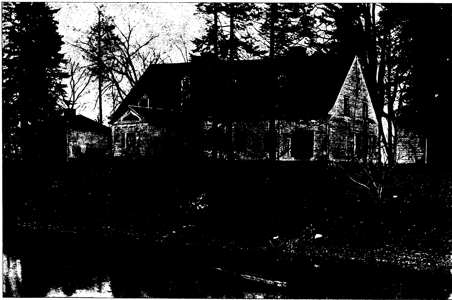
THE BERTHIER MANOR HOUSE—VIEW FROM RIVER.
