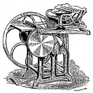
These Presses are all built with the latest improvements, and of the latest s'yle introduced by the Inventor. the Quarto and Half Medium, in combination with the Ink Distributing Table above the form, are used a Cylinder, a Vibrating Feed Roller, and a Fountain, below the form.
