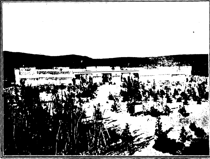
MEXICO—FACADE OF A PALACE IN THE RUINS OF MITLA.
