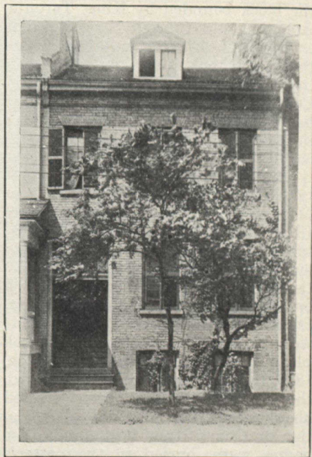
House still standing at 82 Bond Street, Toronto. It was presented by friends in 1858 to William Lyon Mackenzie, and occupied by him until his death in 1861
