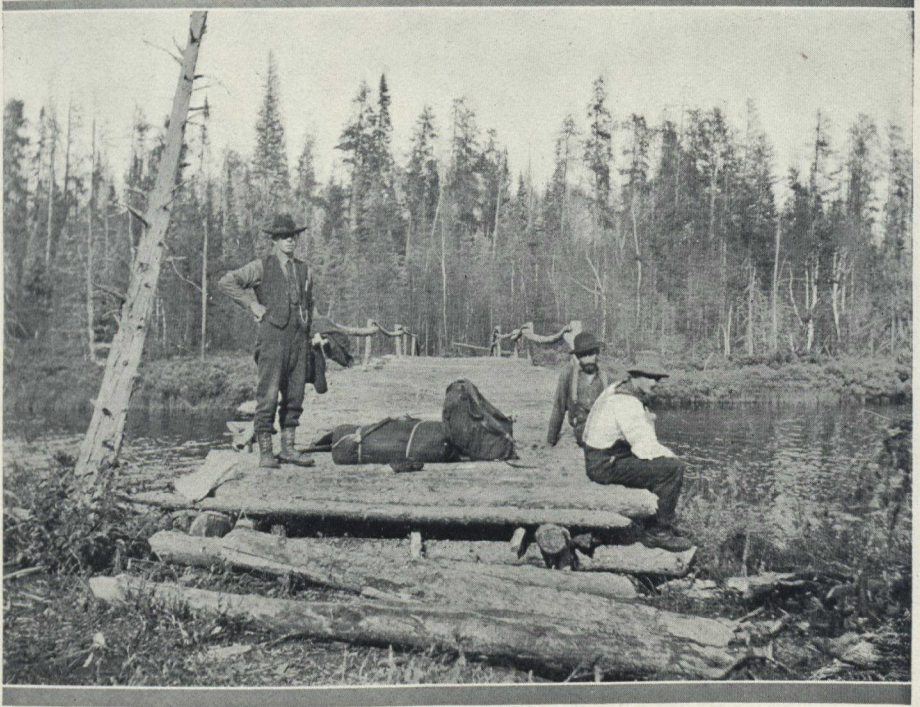
A CORDUROY BRIDGE ON THE ROAD TO GOWGANDA
