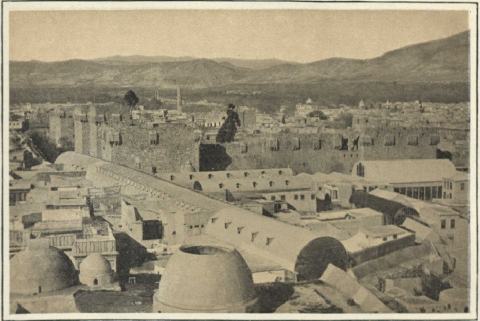
VIEW SHOWING ROOFS OF BAZAARS AND OLD CITADEL, DAMASCUS
