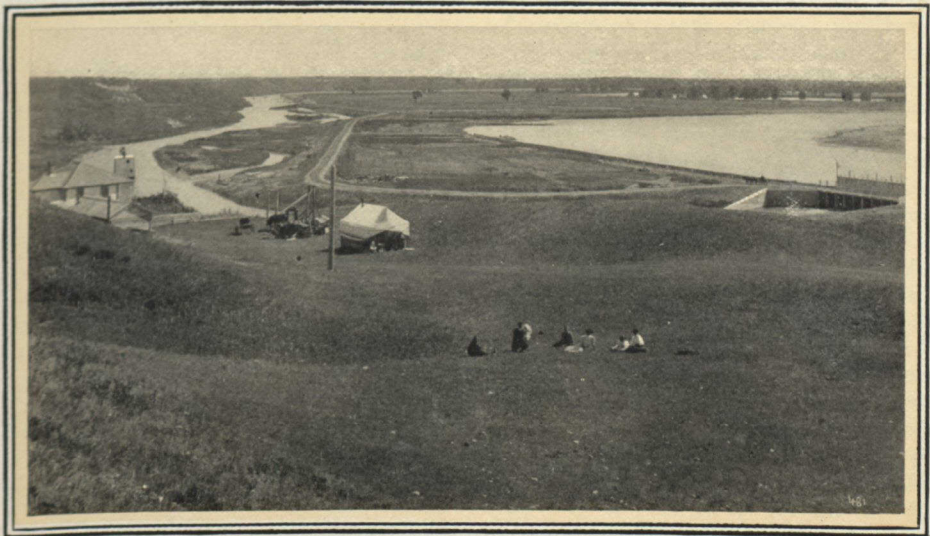
A VIEW OF THE CANADIAN PACIFIC RAILWAY IRRIGATION WORKS, NEAR CALGARY
