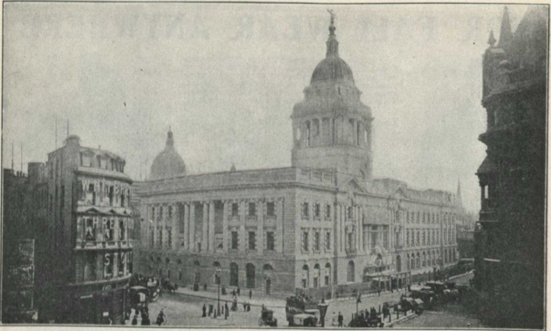
The new Bailey is worthy of the greatness of modern London and takes rank with the great palaces of justice for which Europe is celebrated. Frontage, 287 ft. (Old Bailey) and 142 ft. (Newgate St.); average height from pavement to top of balustrade, 75 ft.; height of dome to the ball, 195 ft.; bronze figure of Justice, 12 ft. high; civic sword held by statue, 6 ft. long. Figures over entrance representing "The Recording Angel," "Truth" and "Fortitude," sculptured by Mr. F. W. Pomeroy, A.R.A.
