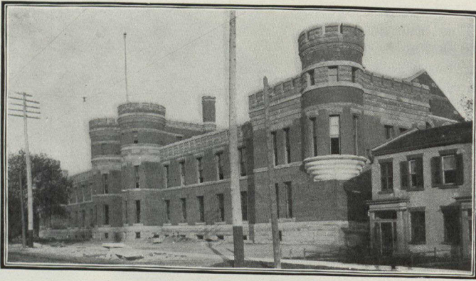
DRILL HALL AT LONDON, ONT.
