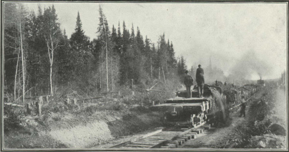
BALLASTING A BIT OF NEWLY-LAID TRACK
