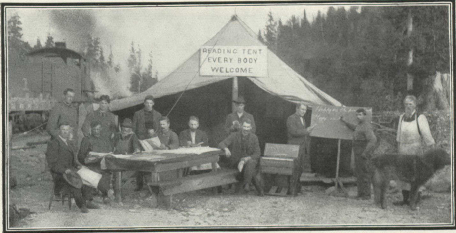
A READING TENT IN A RAILWAY-CONSTRUCTION CAMP, ONTARIO
