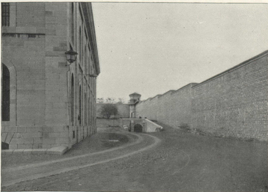
KINGSTON PENITENTIARY—THE WALLS FROM THE INSIDE. THESE WALLS WERE BUILT IN 1845
