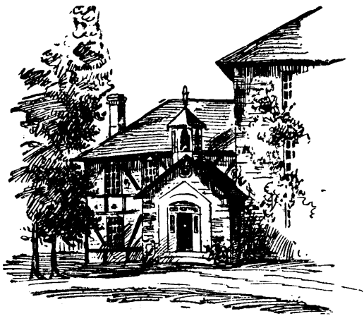
WING OF SHINGWAUK HOME.
