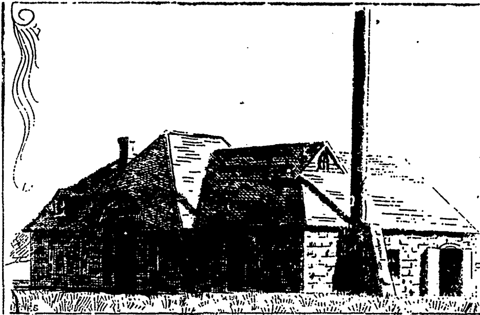
CALGARY WATERWORKS PUMPING STATION
