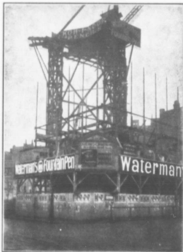
Koh-I-Noor House, London, in Course of Construction.
