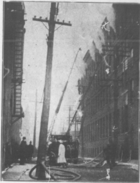
WHERE THE BULK OF CANADA'S HEAVY FIRE LOSSES OCCUR Between 70 and 80 per cent of the national fire loss takes place in factories, warehouses and other high-value mercantile buildings.
