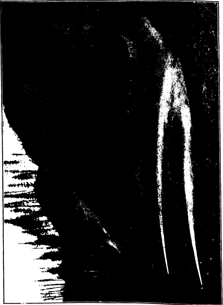
PAIR OF GIANT 7-INCH NOZZLES AT WORK AT CARIBOO HYDRAULIC MINE.
