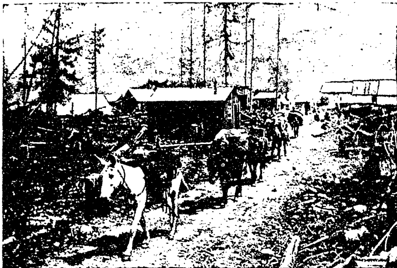
PACKING SUPPLIES TO THE MINE.
