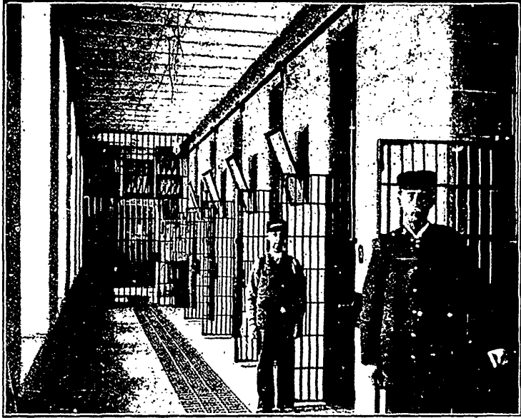
A CORRIDOR WITH CELL DOORS OPEN.
