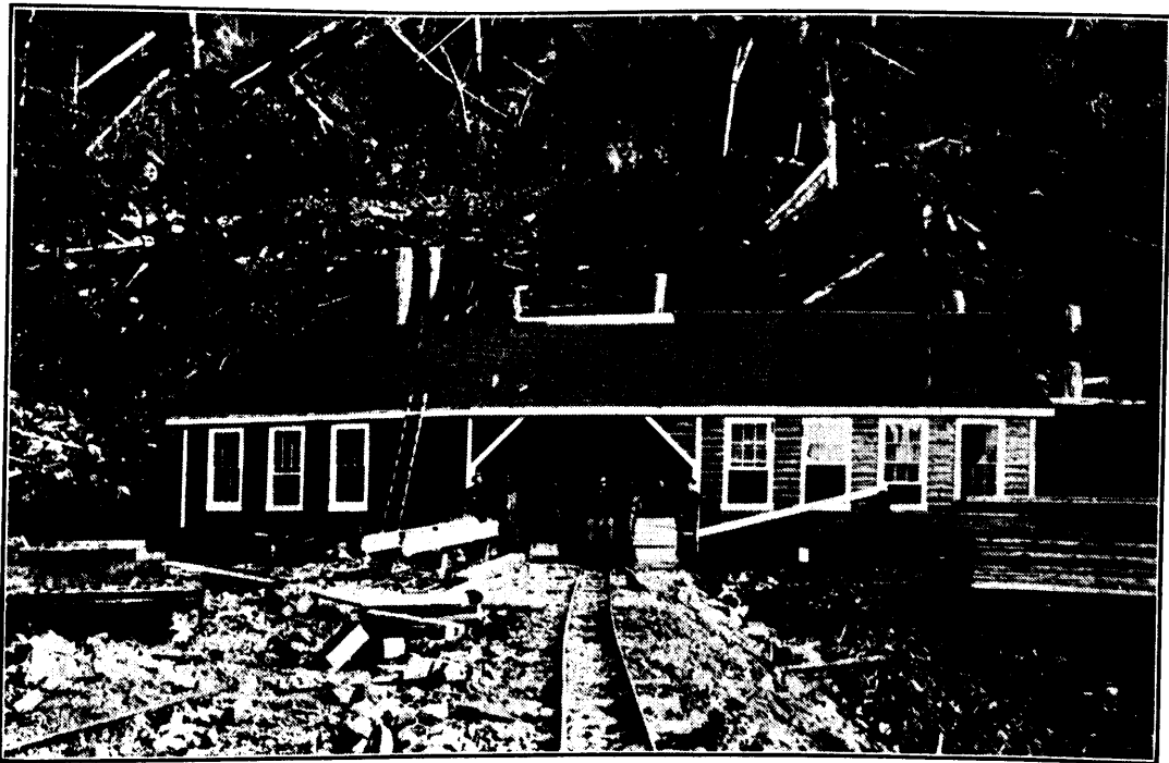
Portal of Cross-cut Tunnel being driven by Rambler Cariboo Mines, Ltd., about half way between McGuigan and the Company's mine, on Dardanelles Creek, Slovan Mining Division. The Tunnel, which is now in about 1,400 ft., will be about 4,300 feet by the time it cuts the vein at a depth of more than 1,400 feet, or 600 feet below the bottom of present 800 ft. main shaft, with which it will eventually be connected by a raise. It is 7 ft. by 7 ft. 6 in. in the clear, with water box 1 by 2 ft. under car track.
