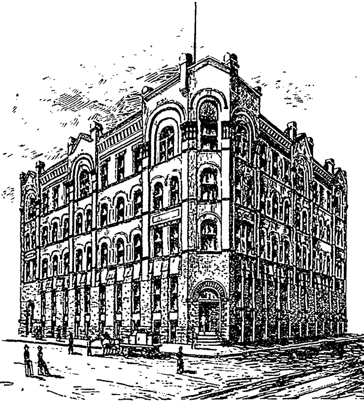
J. W. PECK & CO'S. NEW WAREHOUSE.
