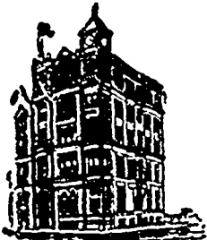
HEAD OFFICE BUILDING, MONTREAL.
