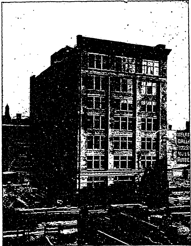
ALLAN WAREHOUSE, TORONTO, ONTARIO. GORDON & HELLIWELL, ARCHITECTS. The entire construction of this building is of Kahn Reinforced Concrete, including footings, columns, girders and floors.
