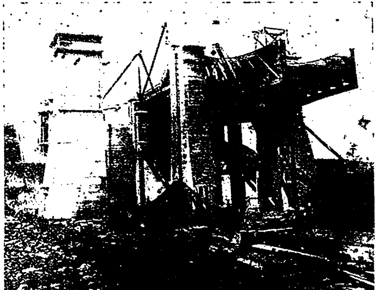
Hydraulic Lift Lock—View from Lower Level.
