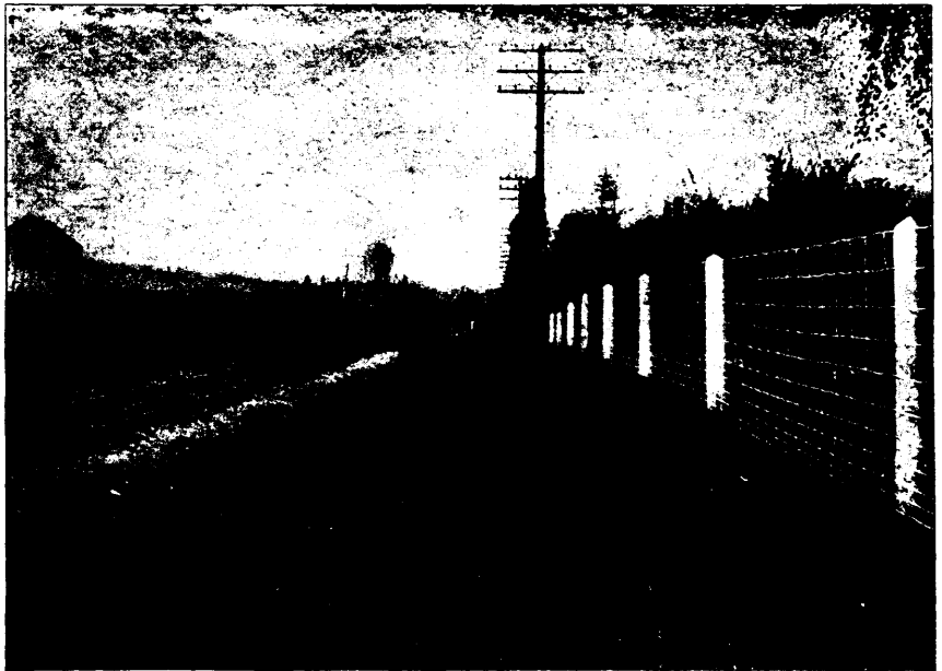
PAGE FENCE ON G.T.R., NEAR SOUTH PARKDALE, ONT.
