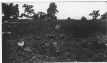
The boulder after the blast.
