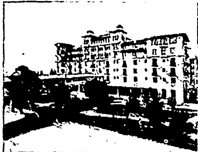
An Absolutely Fireproof Building Completed in 1898.
