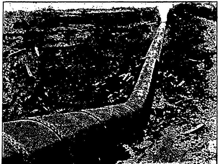
FIG. 4.—CATARACT POWER COMPANY—PIPE LINE, SHOWING HEEL.
