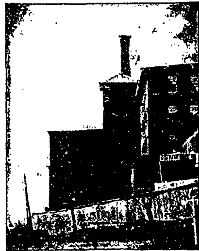
FIG. 3.—THE SAME CHIMNEY AFTER THE AMERICAN STOKER WAS INSTALLED.
