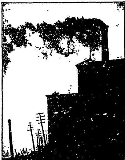
FIG. 2. PHOTOGRAPH OF CHIMNEY BEFORE THE AMERICAN STOKER WAS INSTALLED.
