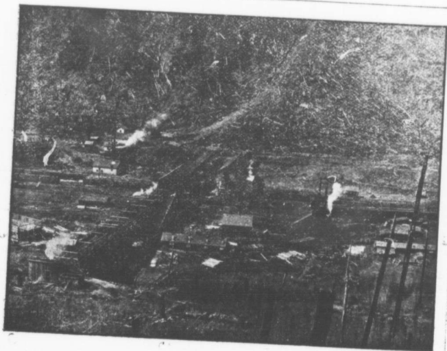
■ At Coal Creek
