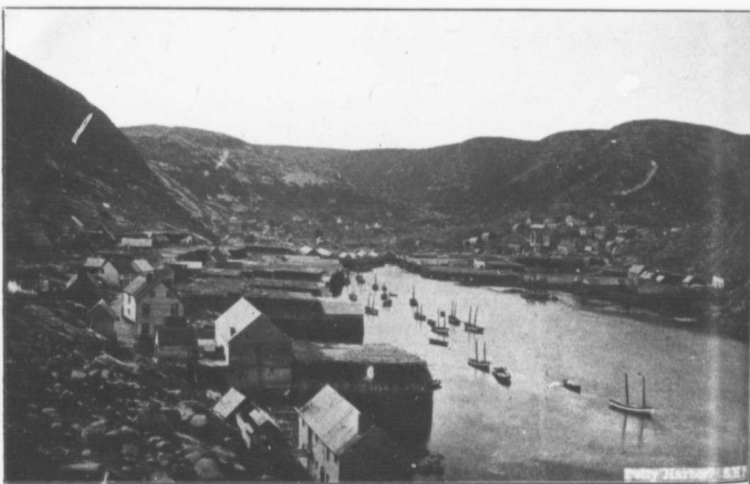
NEWFOUNDLAND—Petty Harbour. The Reid Newfoundland Company's power plant is located here.
