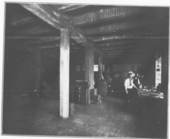
The new warehouse of the Otto Heineman Phonograph Supply Co., showing packing and shipping department.
