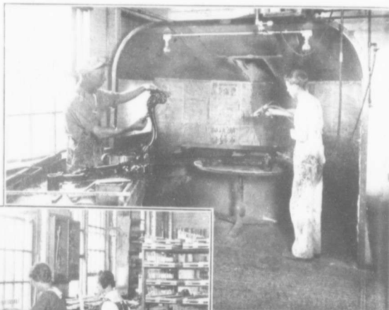
Top—The old and the new way of spreading varnish. The man gets the old brand, does work of three men by the old method.
