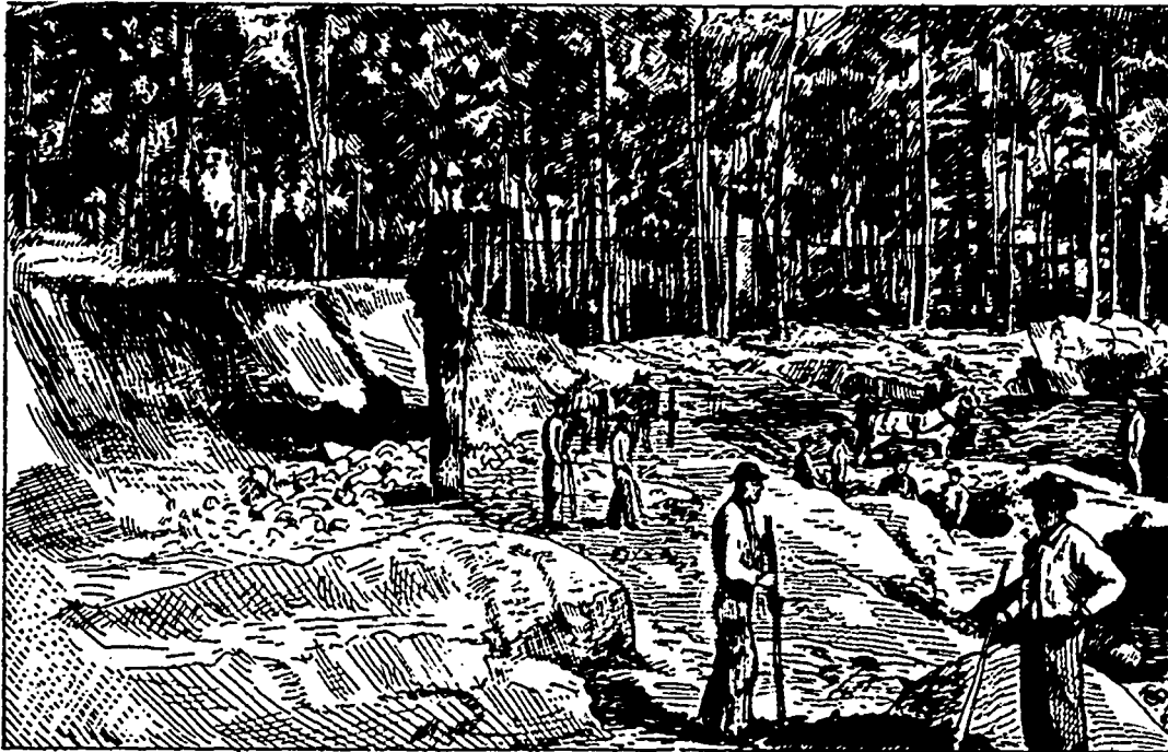
EXCAVATING LAND PHOSPHATES, FLORIDA.
