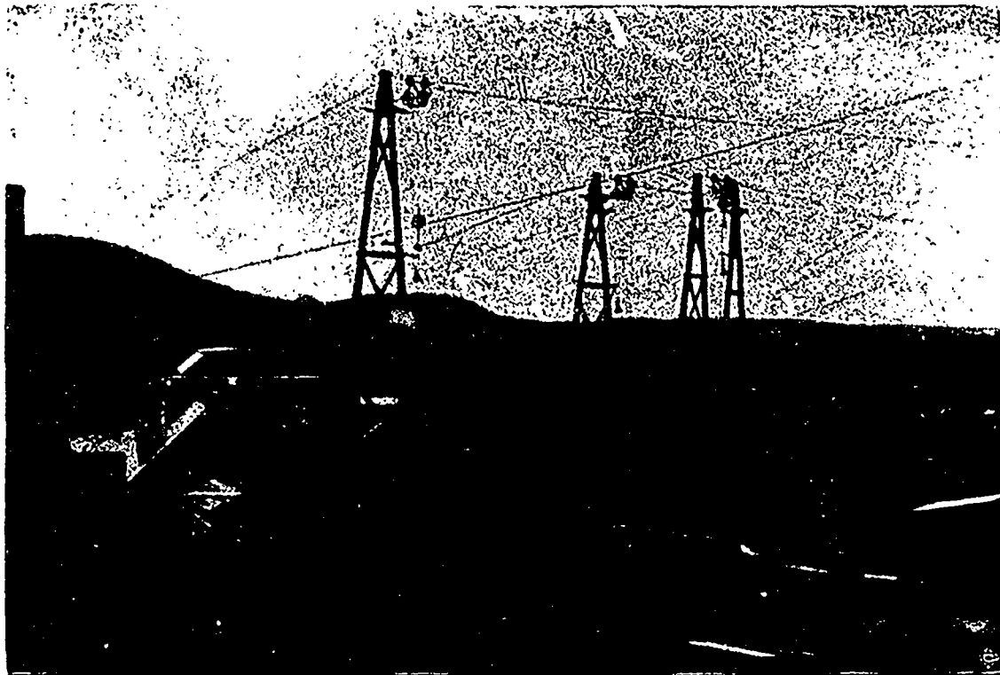
Cable Derricks and Surface Plant at Danville, Que., operated by the Asbestos and Asbestic Co. Ltd.
