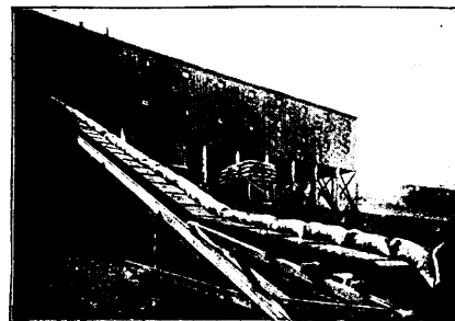
Freight and Package Elevator
