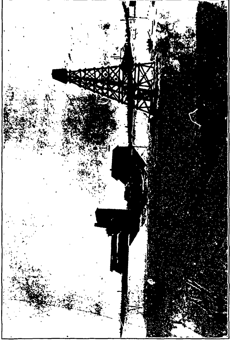
New Reduction Works of the Ottawa Gold Milling and Mining Co., at Keewatin, Ontario, showing Locke-Miller Cableway, crossing railroad, for taking ore from lake barges to sampler.
