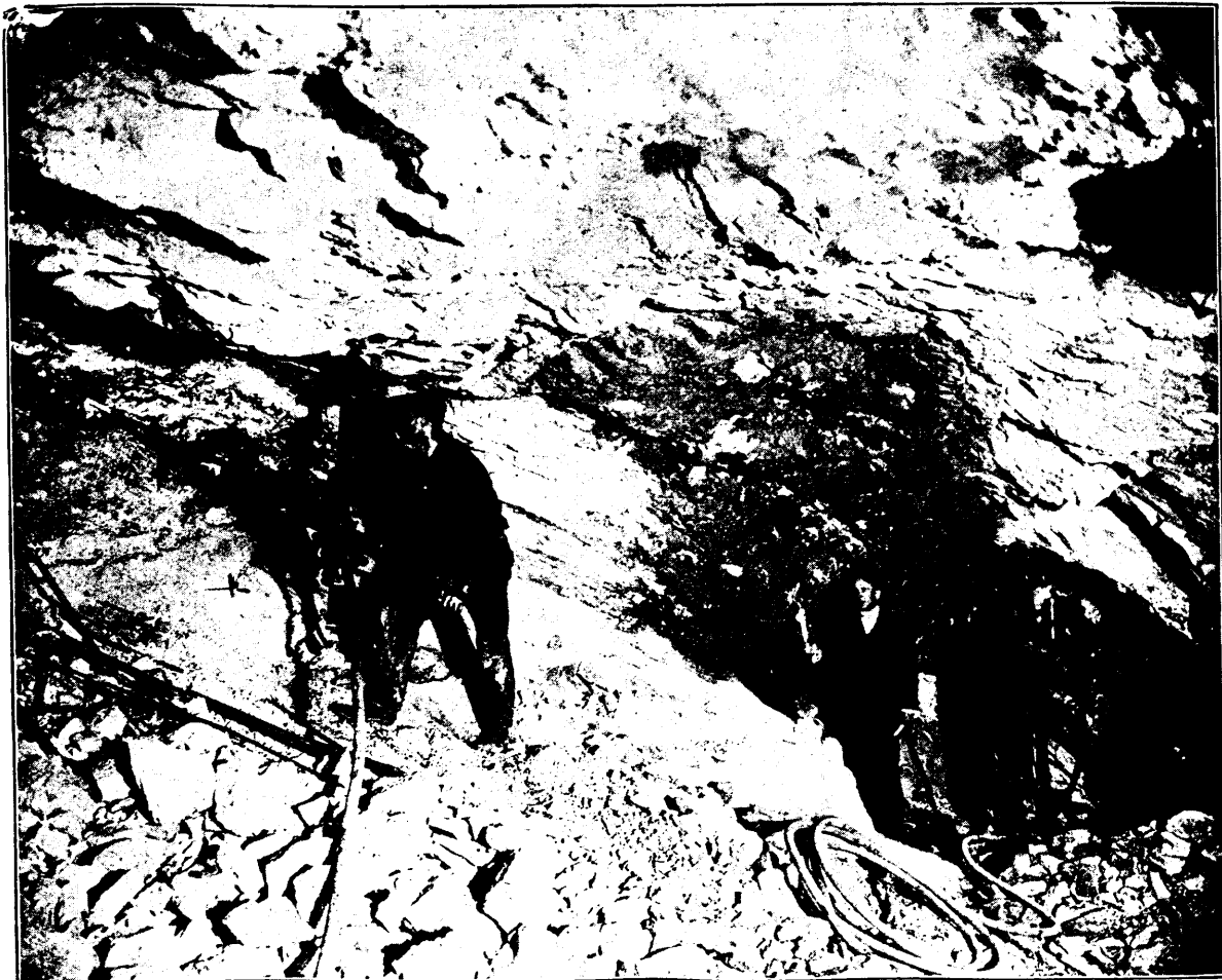
Two 2½-inch Sullivan Drills working on 900-foot level of the Congress Mine, Congress, Arizona.
