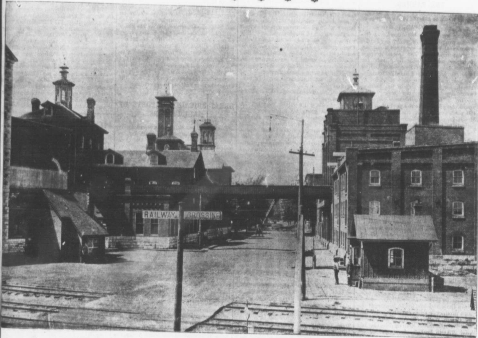
VIEW FROM THE RAILWAY LOOKING NORTH.
