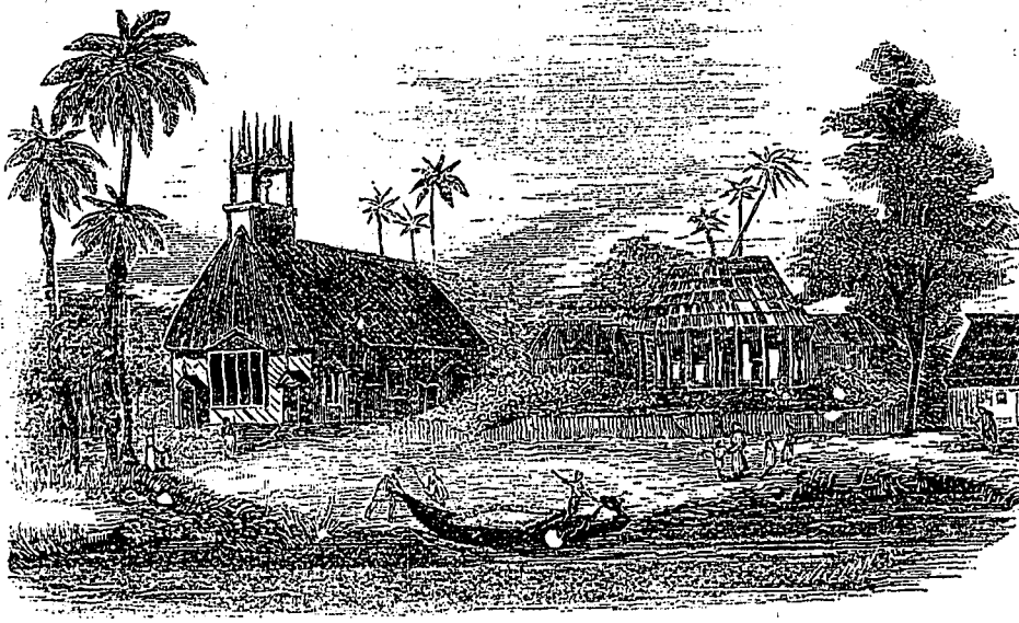
SCHOOL-HOUSE AND CHAPEL AT MBUA FIJI.
