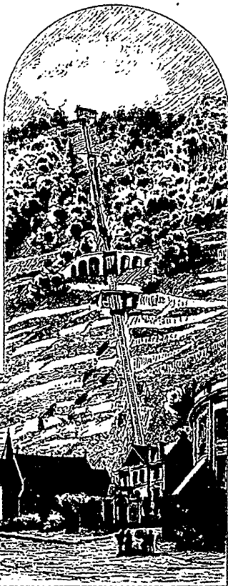
CABLE RAILWAY AT TERRETET-GLION.
