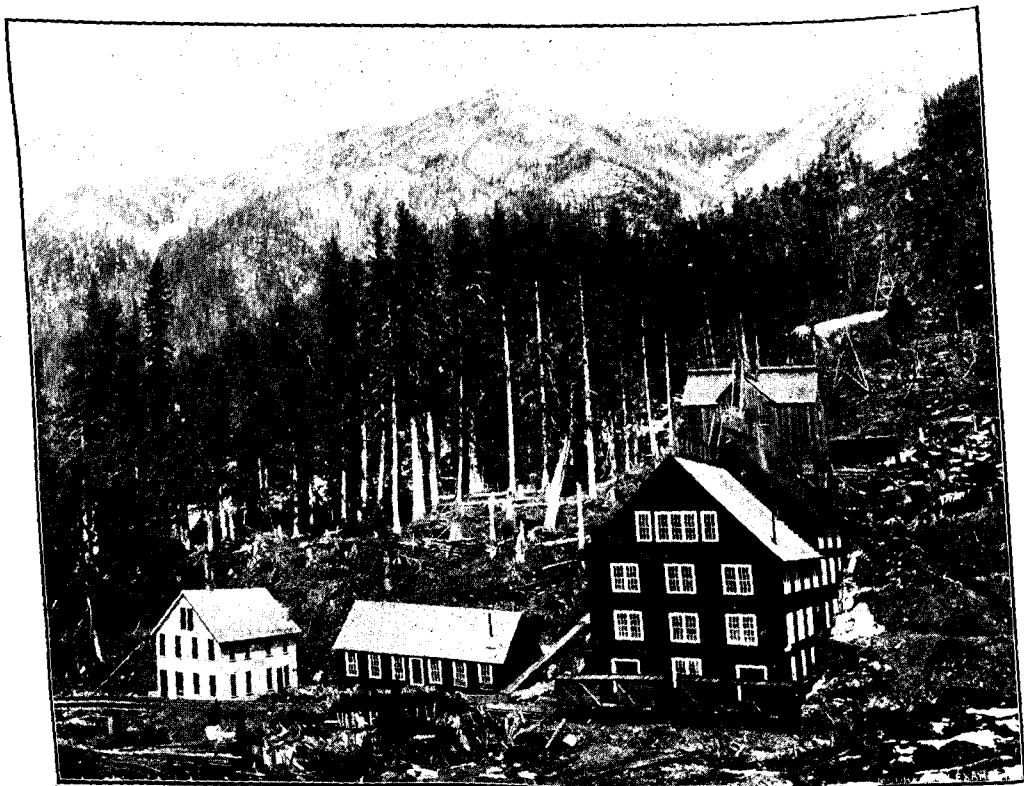
CONCENTRATOR PLANT, NOBLE FIVE.
