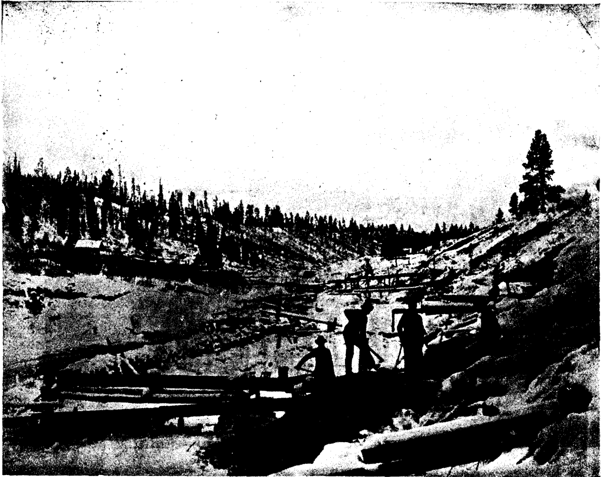
Atlin—Sluicing on Pine Creek, Nov. 30th, 1899.
