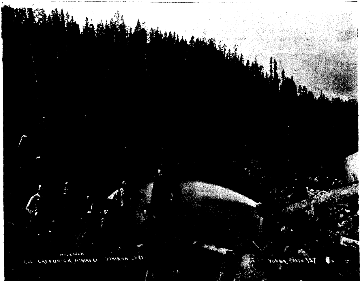
Atlin—Mining by Hydraulic Process on Dominion Creek, a Tributary of Spruce.
