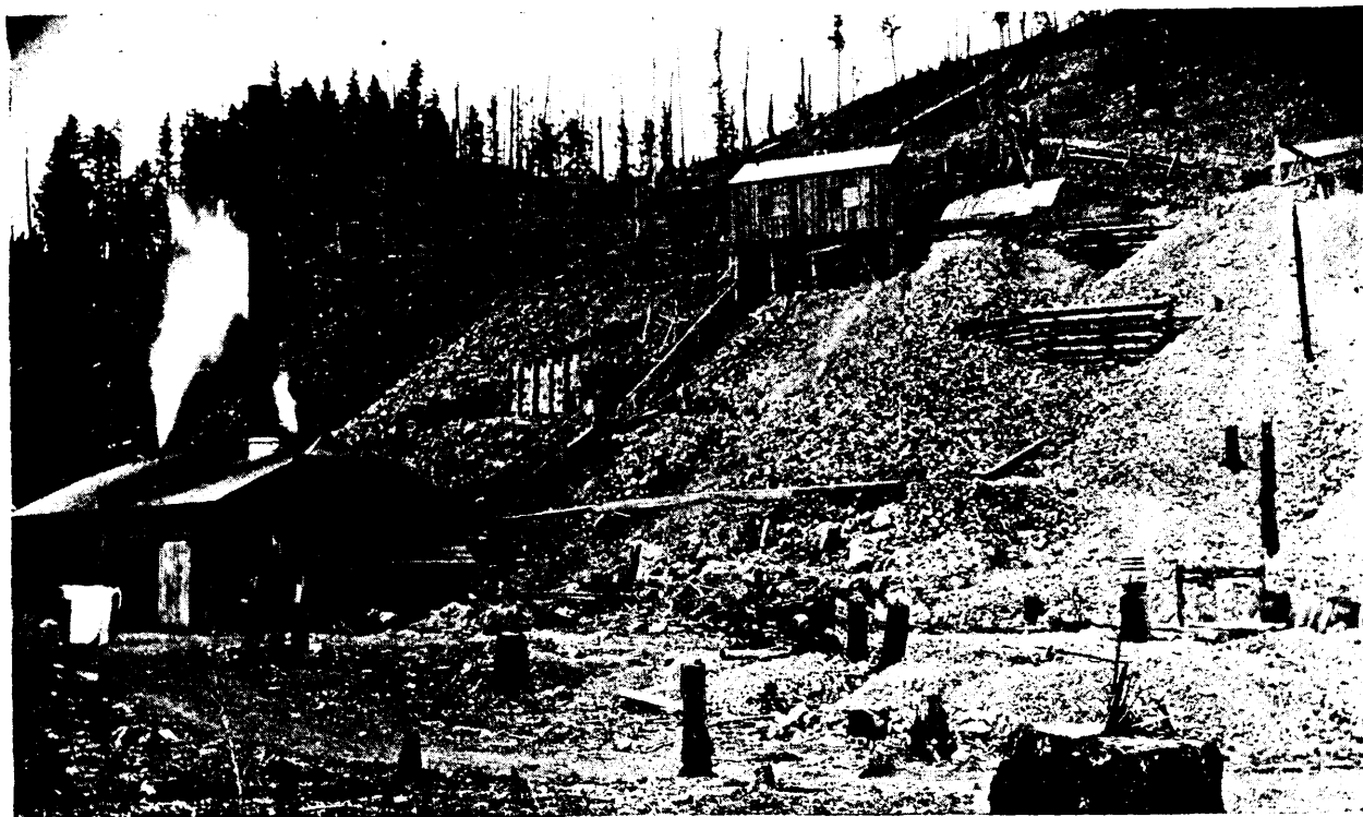
General View of Works.
