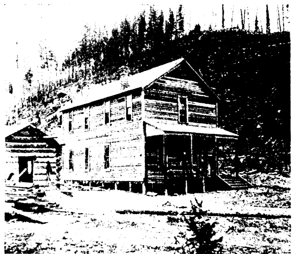
Men's House—Nearing Completion.
