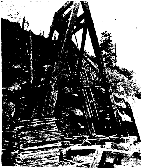
Building Gallows Frame.
