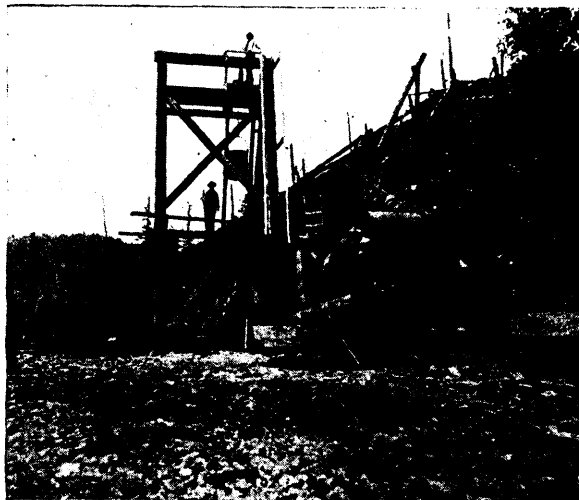
Gallows Frame and Hoist in Position.
