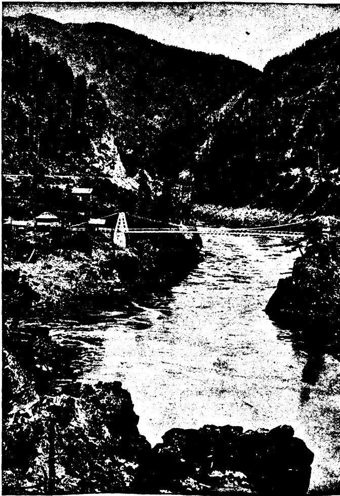
FRASER RIVER, WITH SUSPENSION BRIDGE.
