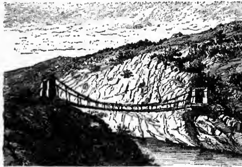
BRIDGE OVER THE RIVER PACHACHACA, MADE OF THE FIBRE OF THE MAQUEY.
