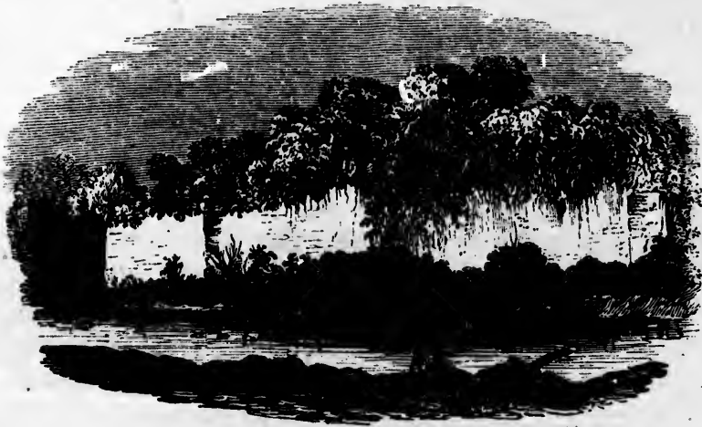
Fig. 29.—Great Wall at Copan.
