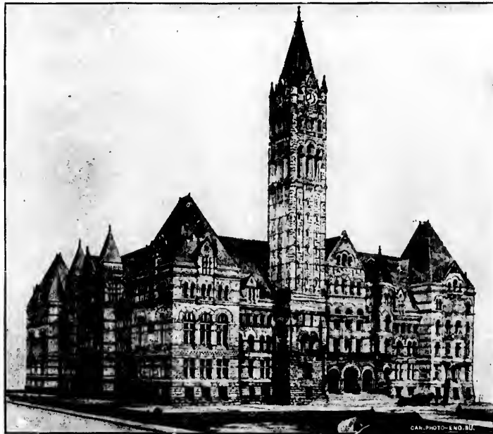
NEW MUNICIPAL AND COUNTY BUILDINGS.
